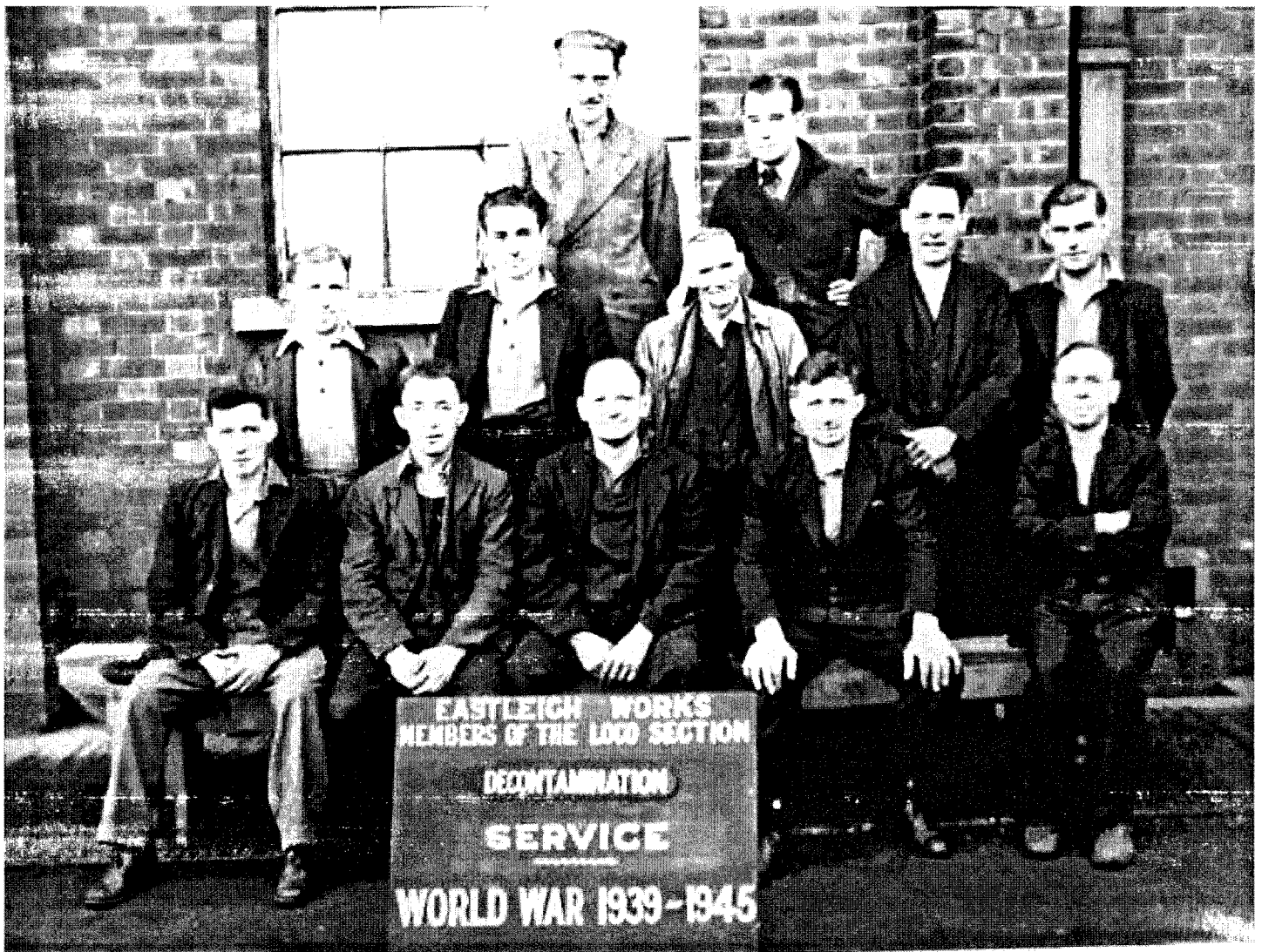
Loco Section of Decontamination Service.
