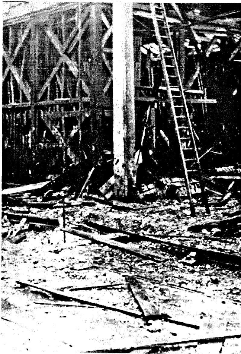
North East Corner of the Iron & Steel Store.
