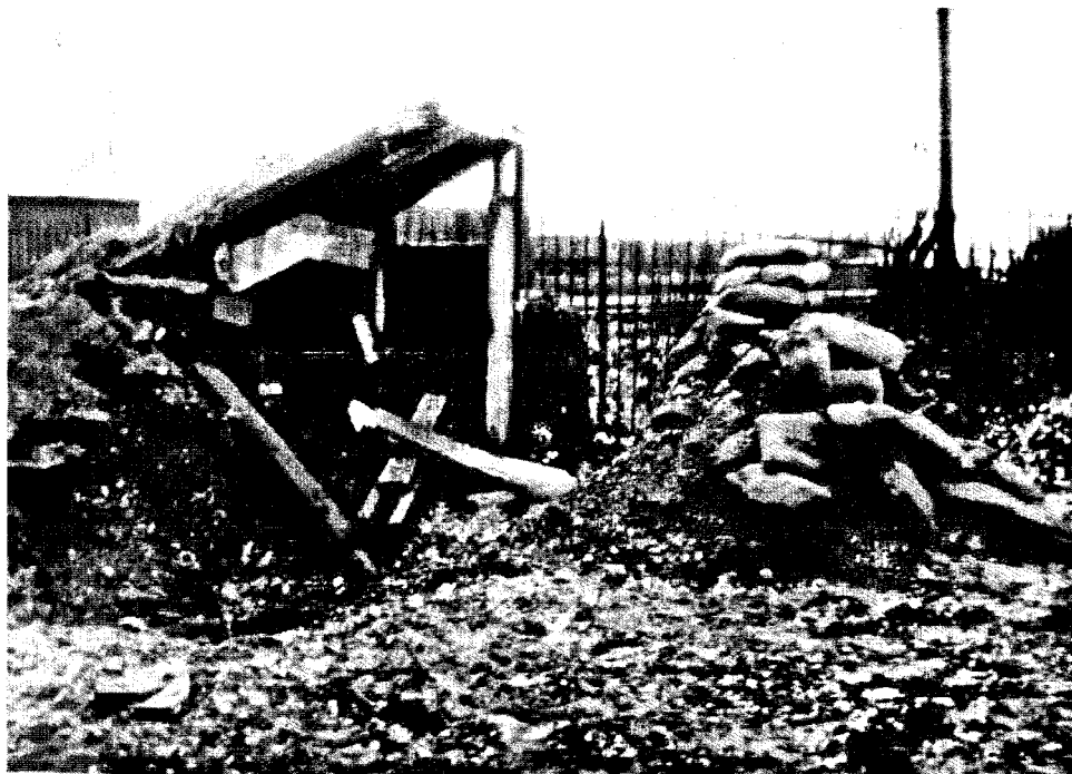
Entrance to Shelter.
