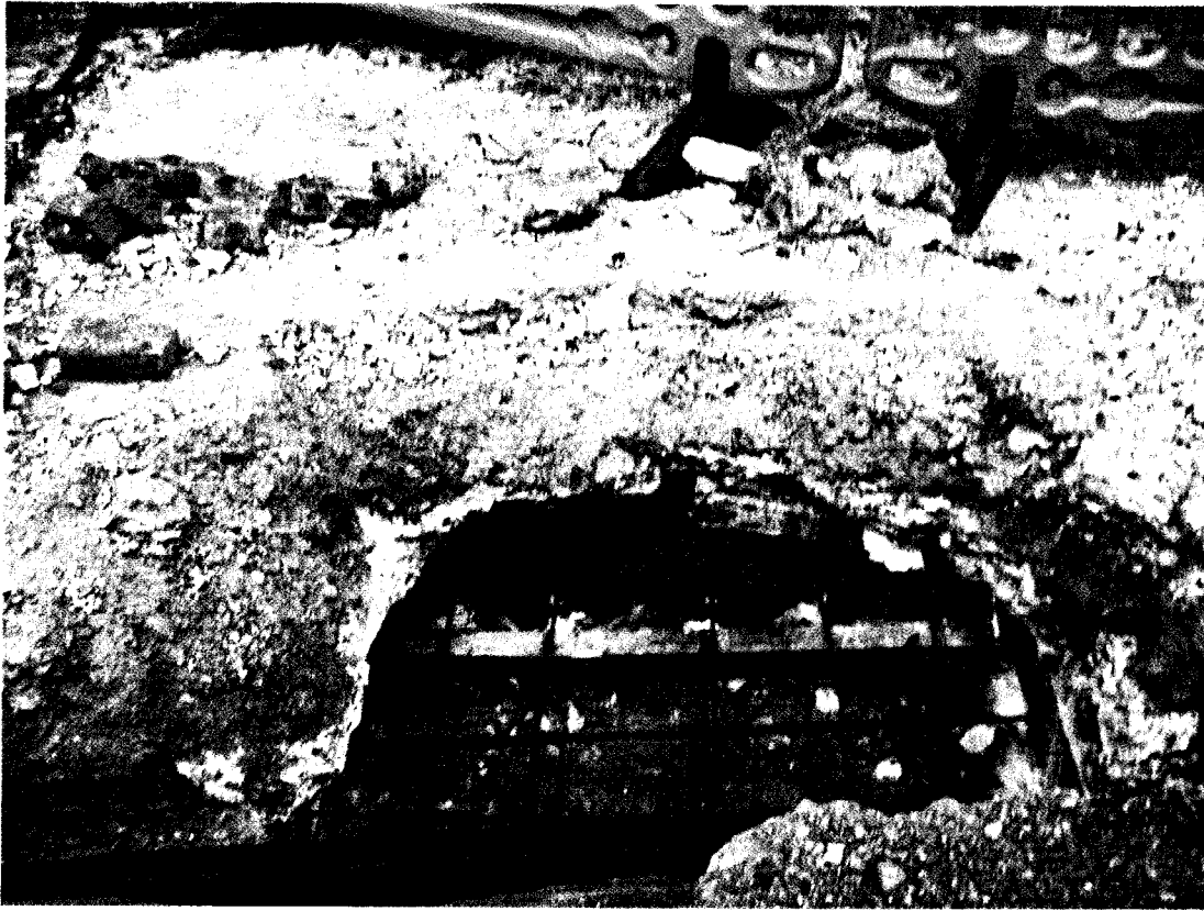
A hole photographed looking east towards the brick Bingo Hall building and about five feet from it near the rainwater pipe. The breeze block wall was probably built during or before the previous demolition. The reinforcement wire grid was placed there in 2015 and is now concreted over. The passage ran from here towards the west.
