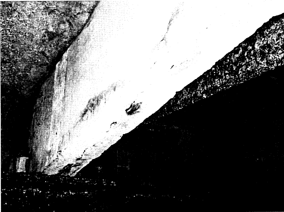
e13. Concrete Spalling – Corrosion of Reinforcement.
