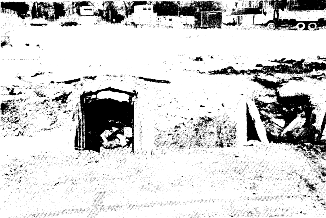
Demolition of the Air-raid shelters in the Recreation Ground, East of the Avenue across the park in February 1983 when Safeways was built.
