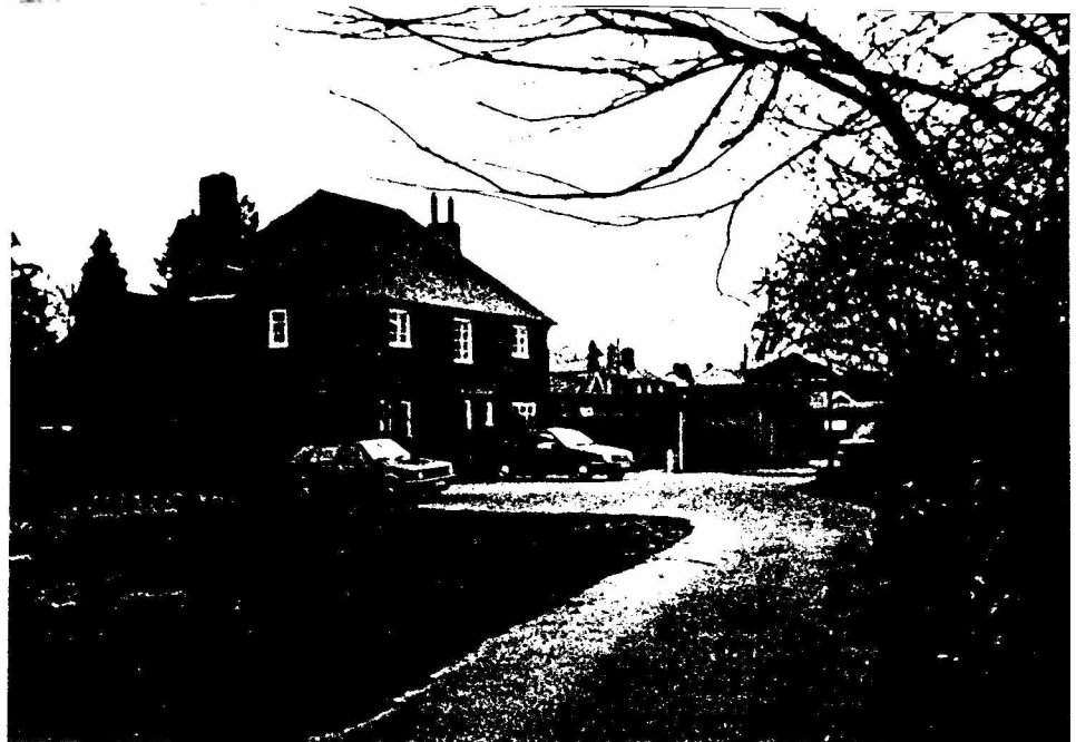
Superintendent's house, 30 Romsey Road.
