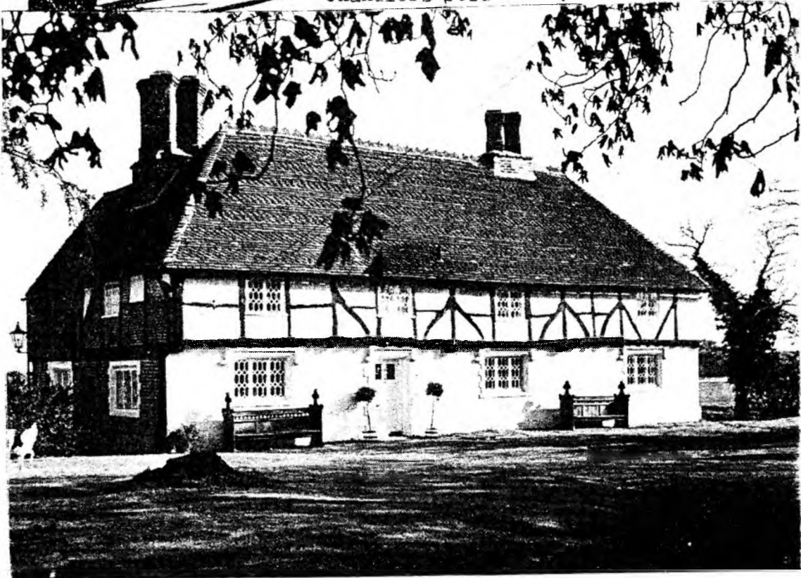
Shamblehurst Manor, Hedge End, an architectural gem.
